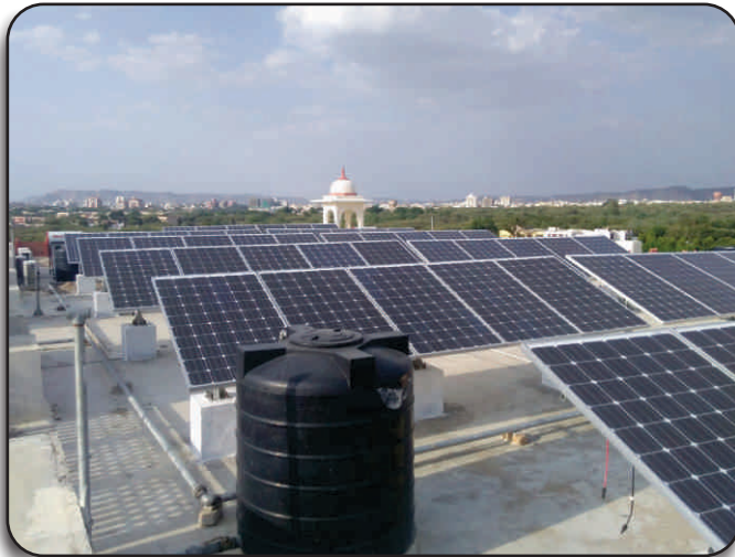
45kWp SPV Grid connected SPV Power Plant installed at RSRDC, jaipur under RREC scheme
